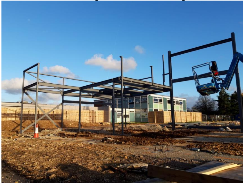
First stages of the new building
